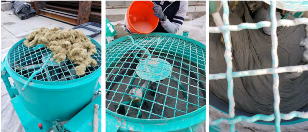
Figure 2.8 UHPC while being mixed in the high shear mixer.
