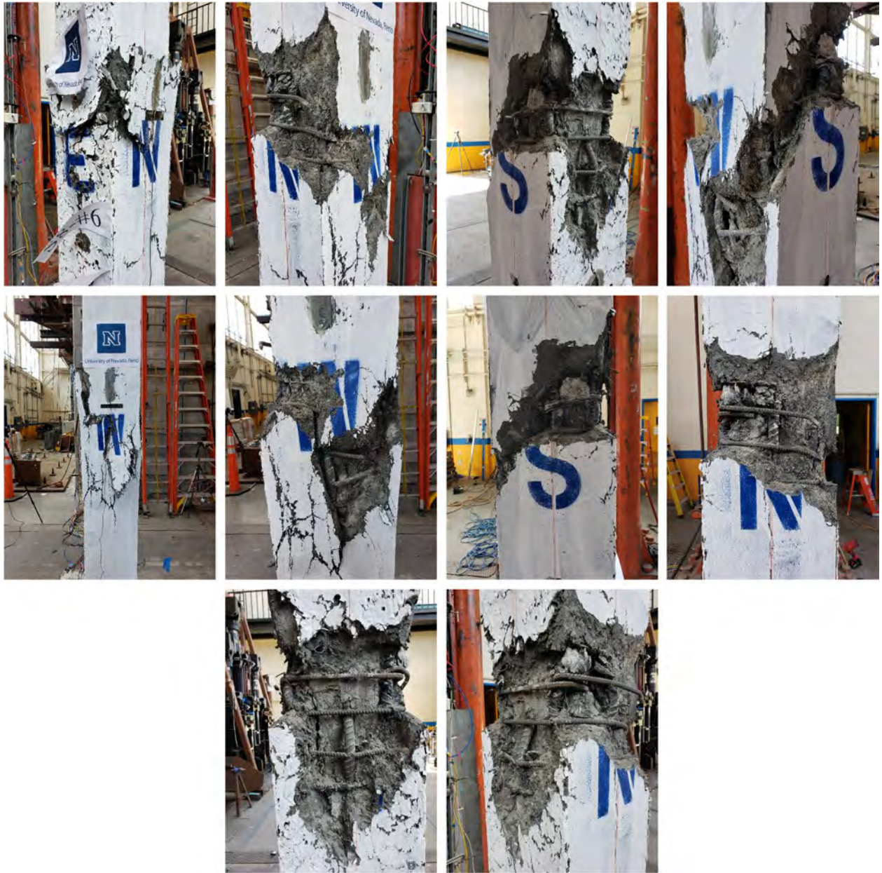
Figure C.8 Final damage state of column S12-L6.
