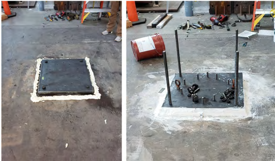
Figure B.13 Placing of the lower plate and hydro-stoning underneath it for leveling.
