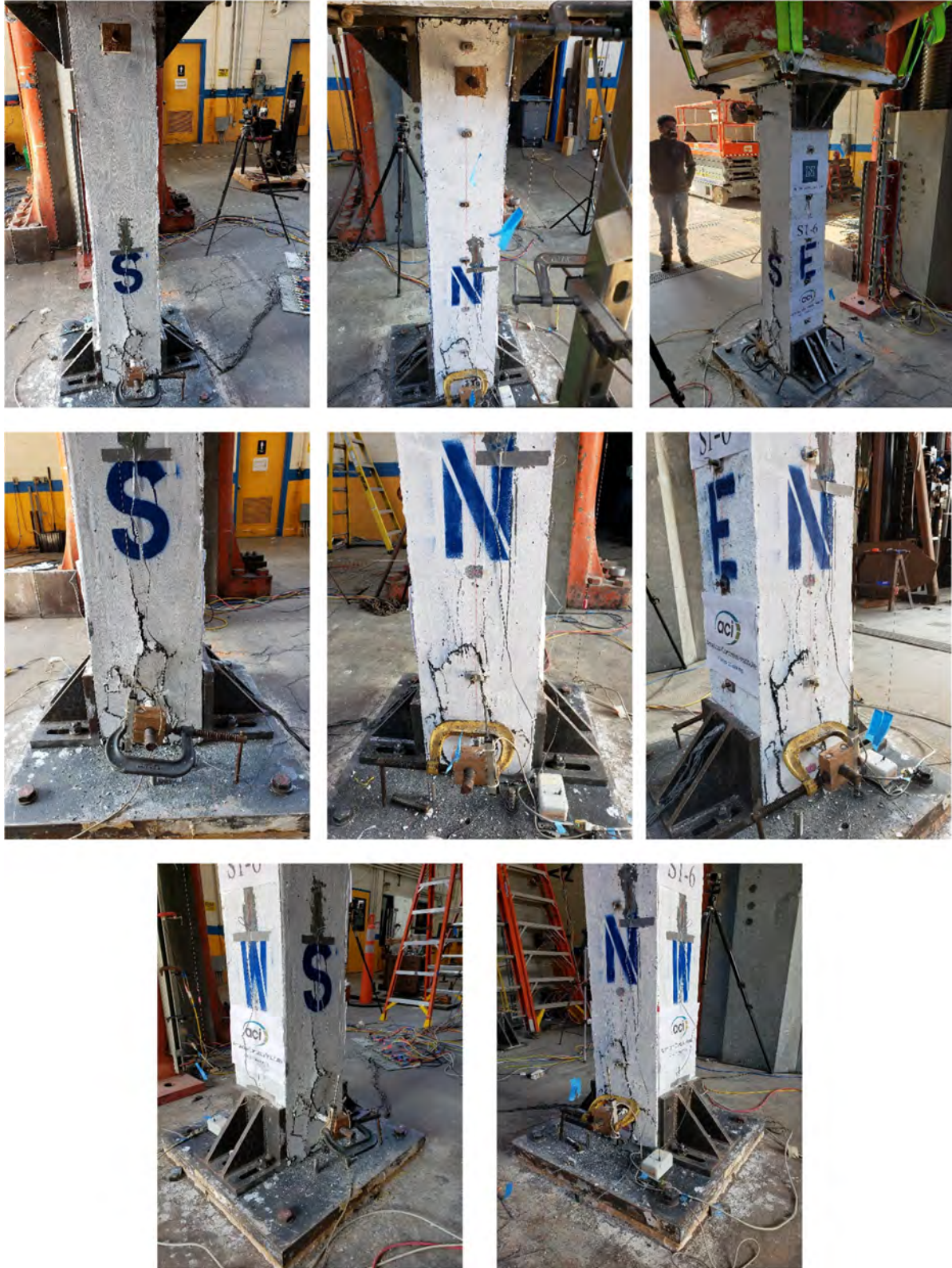
Figure C.1 Final damage state of column S6.
