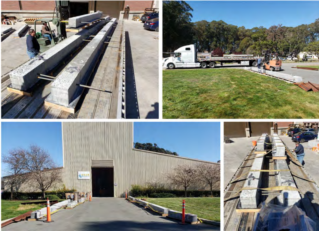
Figure B.10 UHPC columns transportation from UC Berkeley Richmond Field Station Lab.
