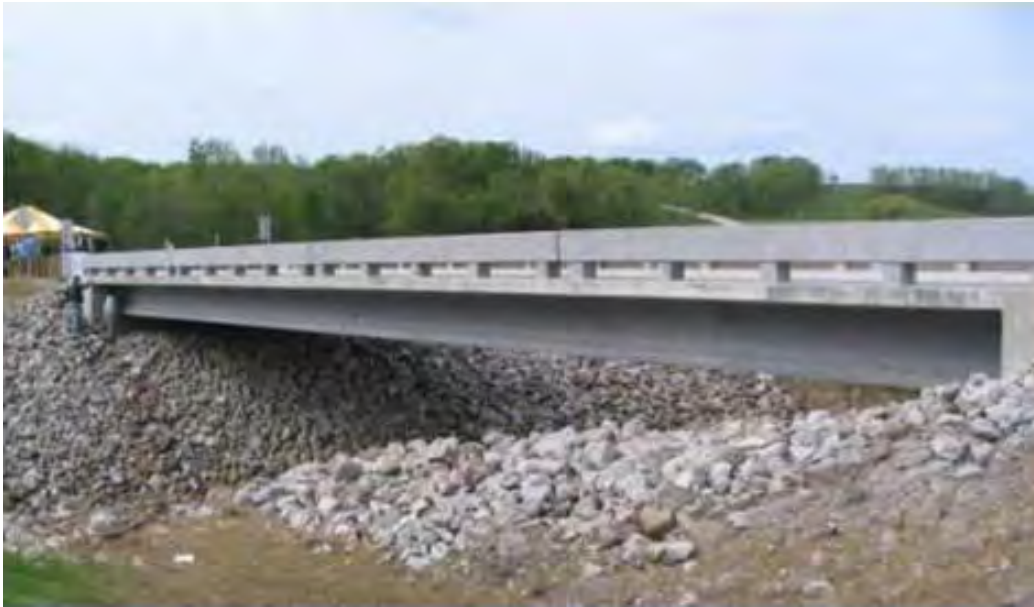
Figure 1.1 UHPC prestressed I-girder bridge in Wapello county, Iowa. Source: FHWA.
