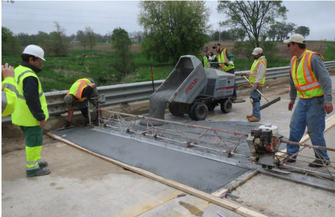
Figure 1.3 Placement of UHPC overlay on the Laporte Road bridge over Mud Creek in Brandon, IA. (Source: Haber et al. 2017).
