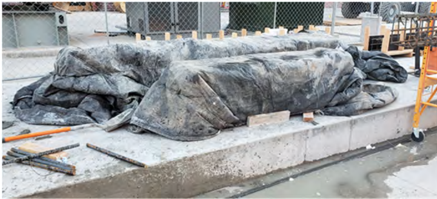
Figure B.8 Use of heat blankets for cast UHPC columns to protect specimens from low temperatures in the Reno area.
