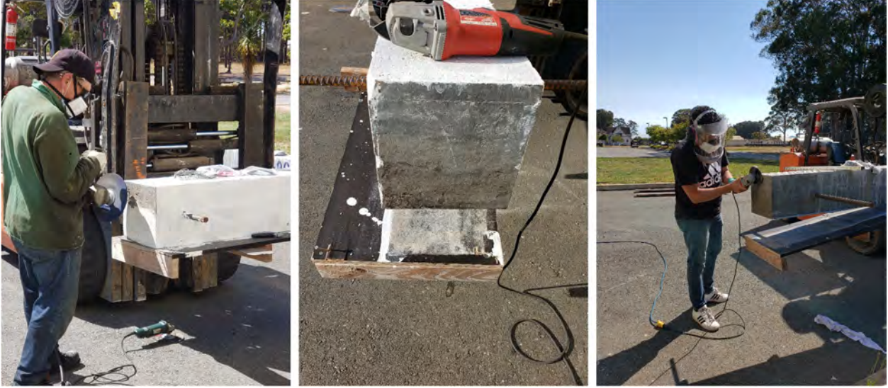
Figure B.15 Grinding of the extra parts at the column ends to make the columns stand leveled.
