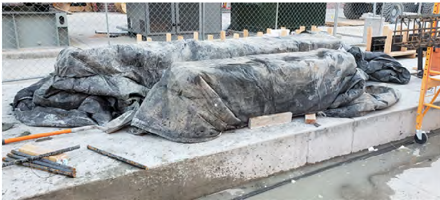
Figure 2.5 Use of heat blankets for cast UHPC columns to protect specimens from low temperatures in the Reno area during winter when the columns were cast.
