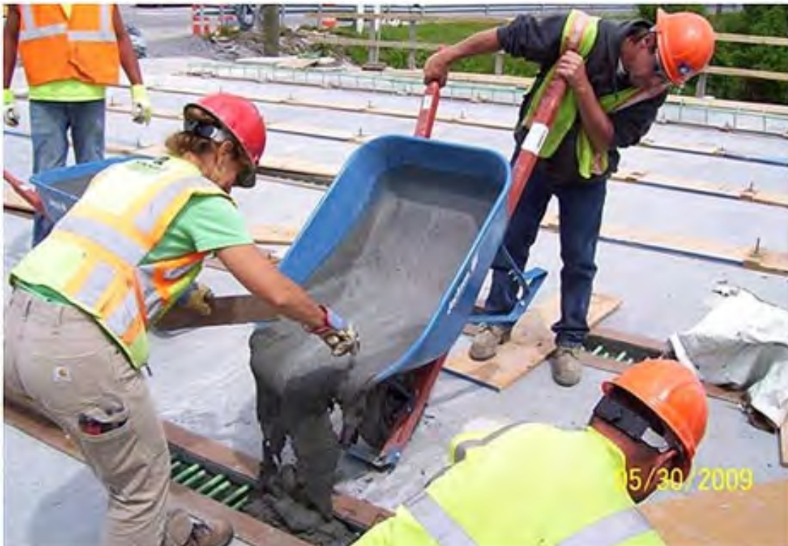
Figure 1.2 Longitudinal field-cast UPC connections between deck-bulb-tee-girders on the Route 31 Bridge in Lyons, NY. Source: New York State Department of Transportation.
