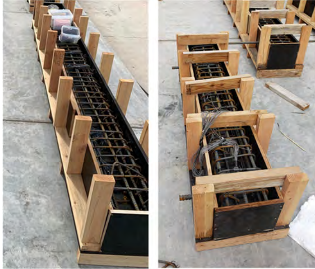
Figure 2.3 Rebar cage as assembled and installed inside the formwork.
