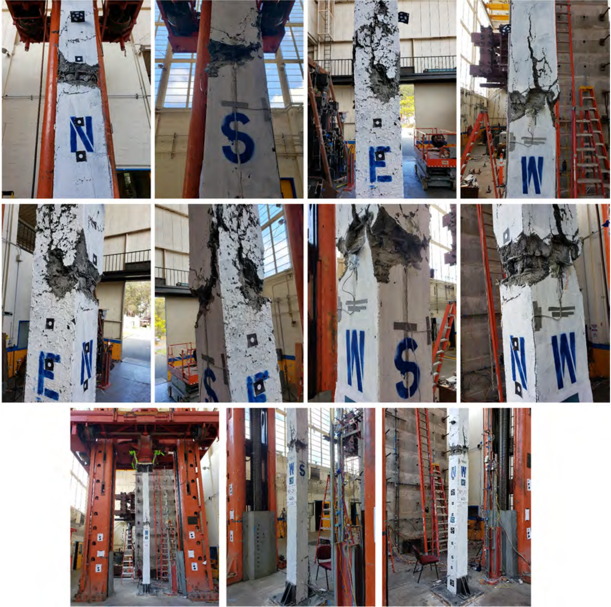
Figure C.5 Final damage state of column S20.
